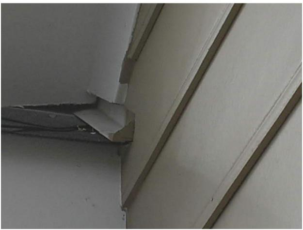
7.8. Black sheathing (builder's felt) is sticking out from under some of the hardboard siding; like on the rear of the garage, and on the left side of the house,
